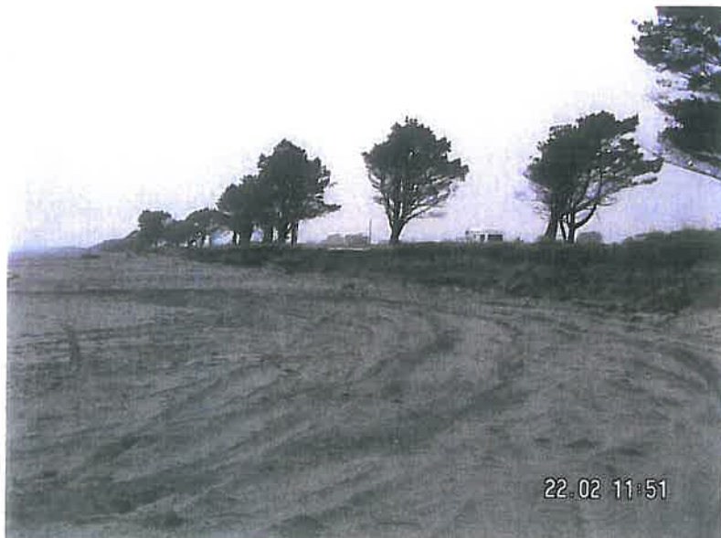
Erosion scarp along Domain Frontage
