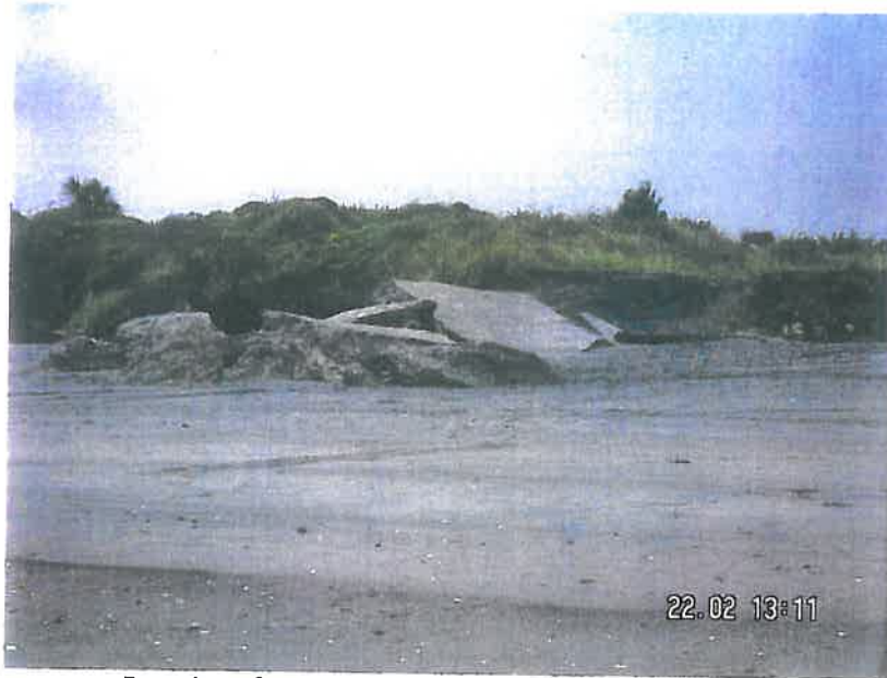
Remains of concrete used to fill accessway blowouts
